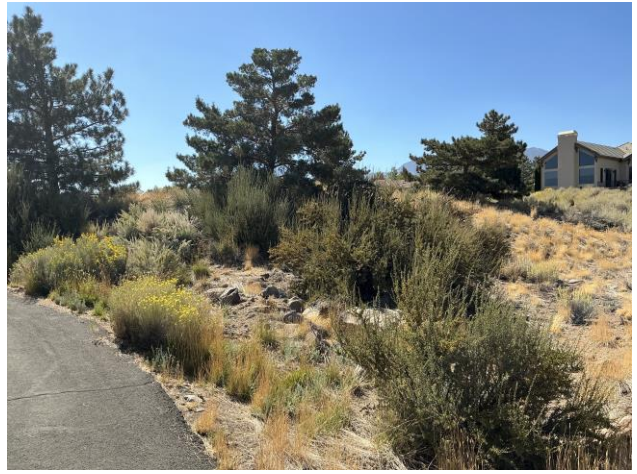
Photo #6 – Tall brush adjacent to planted trees. I recommend creating a “halo” around the trees drip line and then remove the lower branches of the trees (latter fuels).
